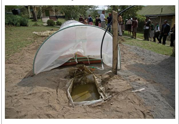
The solution might, in part, come from the use of biogas digesters (shown above). The biogas digesters use any bio-degradable material e.g. animal or human waste, garden weeds and kitchen waste. They are highly efficient, have a life span of over 10 years and come in varying sizes.
